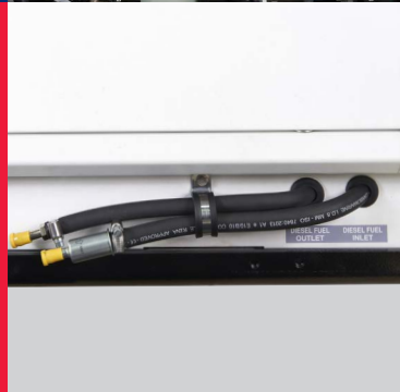
Input/Output fuel pipe
