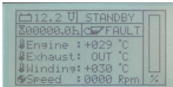
Fig. 15.2-1: Fault: „Cylinder head temperature out of range“
