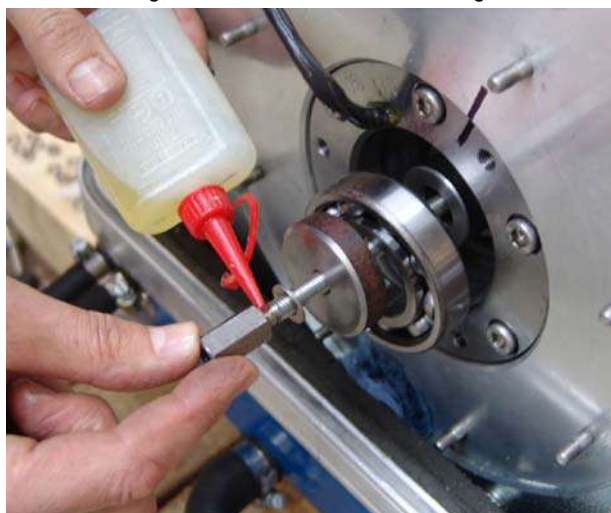
Fig. 7.12.2-26: Mount the ball bearing
