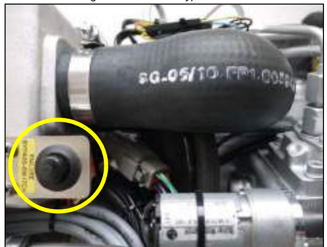
Fig. 6.3.6-5: Failure Bypass switch
