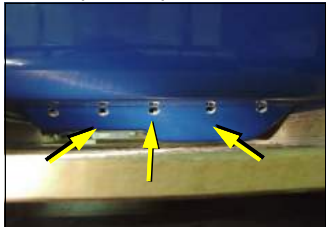
Fig. 6.3.4-2: Drilling for Combustion Air
