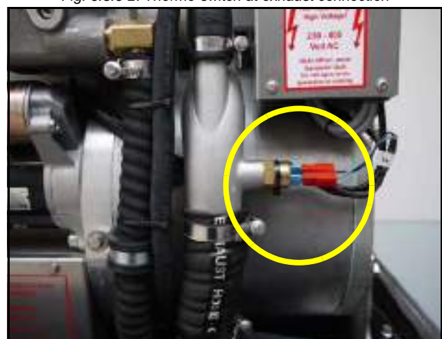
Fig. 6.3.6-2: Thermo-switch at exhaust connection
