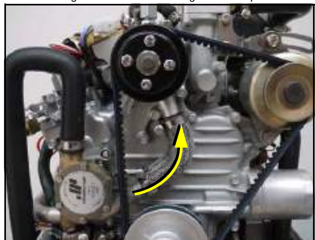
Fig. 6.3.2-6: Internal Cooling Water Pump
