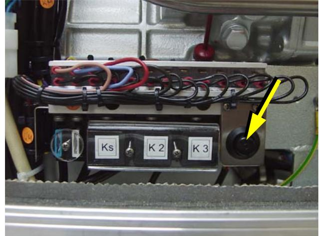
This period can be reduced by pushing the button on the front of the generator. The generator can be started by means of the remote control as long as the button is depressed. The switch/button bypasses any faults allowing the generator to run.
