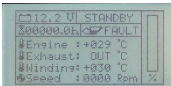
Fig. 16.2-1: Fault: „Cylinder head temperature out of range“
